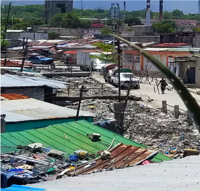
Figure 5. View from rooftop at SAKALA. The canal is completely clogged with trash.
