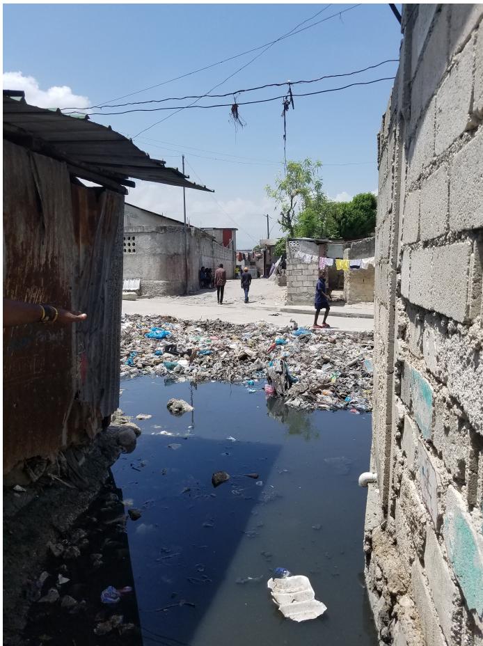
Figure 7. Contaminated water from trash-filled canal rises to SAKALA's back door
